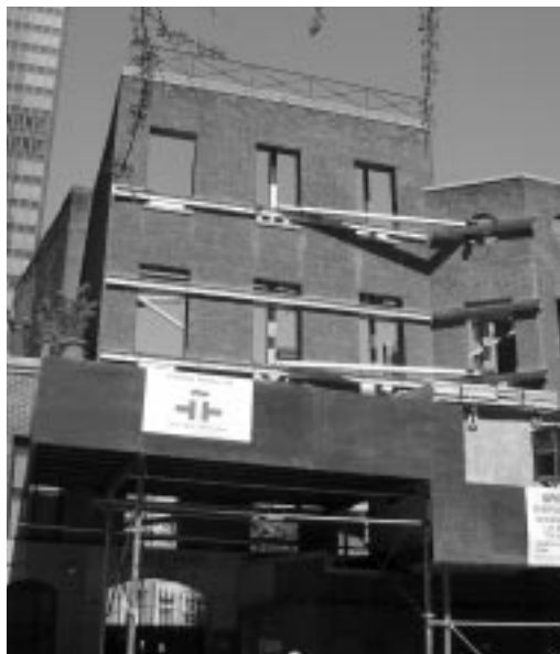
Construction is underway at Amster Yard, and the new cultural center will incorporate its historic façade.
