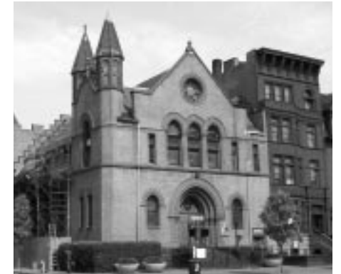
Ebenezer Gospel Tabernacle has installed a new slate roof and copper cladding on the dormer windows, in addition to restoring the stained glass windows and the terra cotta tile on the tower, with help from the Upper Manhattan Historic Preservation Fund.
