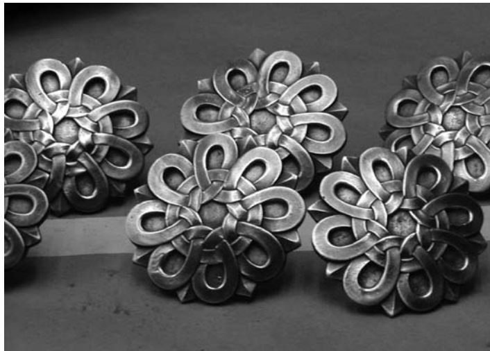
Rosettes on Manhattan’s Temple Emanu-El vestibule wall were removed and restored to match their original appearance.
