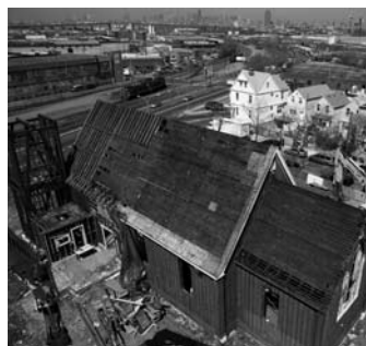
Left: Unfortunately, narrow street widths and overhead bridges and utilities precluded moving the church to its new site without first dismantling it.
