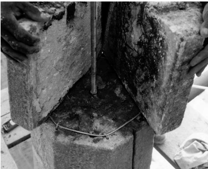
The finials were disassembled and reconstructed with new stainless steel reinforcing.
