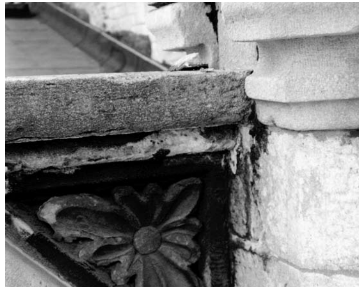
Floral motif with gypsum crust and staining, prior to cleaning.
