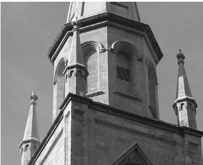
The reconstructed finials
