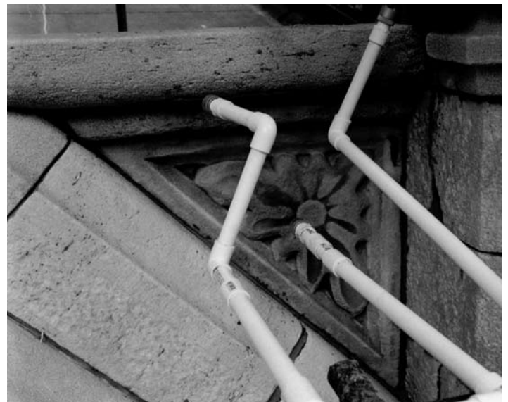
Numerous cleaning tests were conducted with different products that minimized water usage. Nothing worked quite as well as water.
