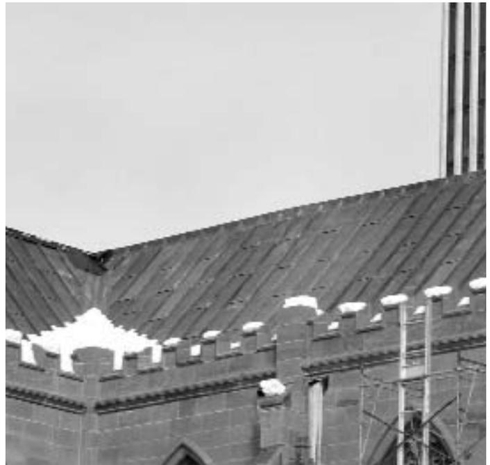
*The Cathedral's lead roofing, drainage system, and re-created crenellated parapets were installed in 2002.*
