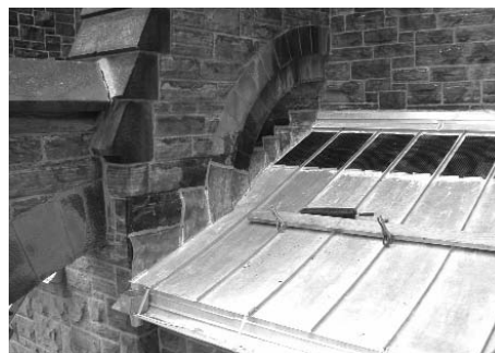
Episcopal Cathedral of All Saints in Albany, NY has a standing-seam, terne-coated, stainless steel roof.
