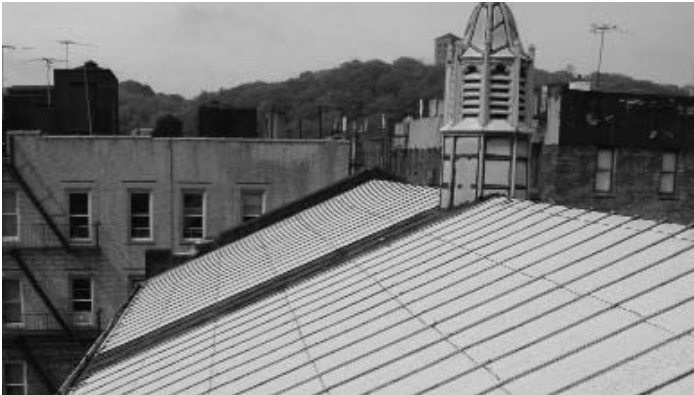
above: Gardner Earl Chapel and Crematorium, Troy, NY has a batten-seam copper roof.
