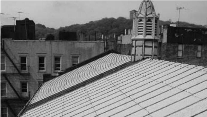
Using the appropriate seam profile is also important. The seam is the type of joinery commonly used to connect metal panels to one another.
