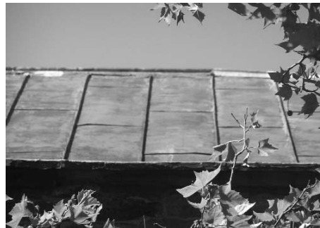
Christ Church in Cobble Hill, Brooklyn, has a standing-seam steel roof.
