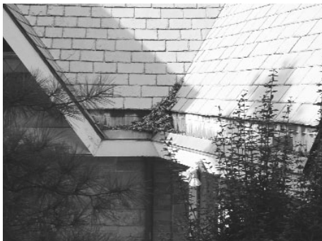
Clean debris from drains, gutters, downspouts and catch basins.
