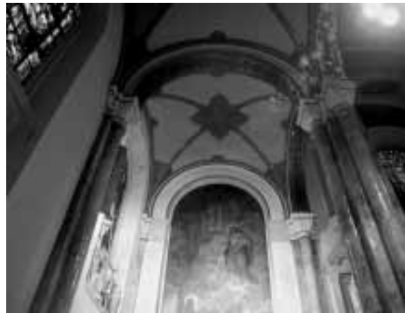
30-ft-high scagliola columns at Roman Catholic Church of the Ascension in Washington Heights.
