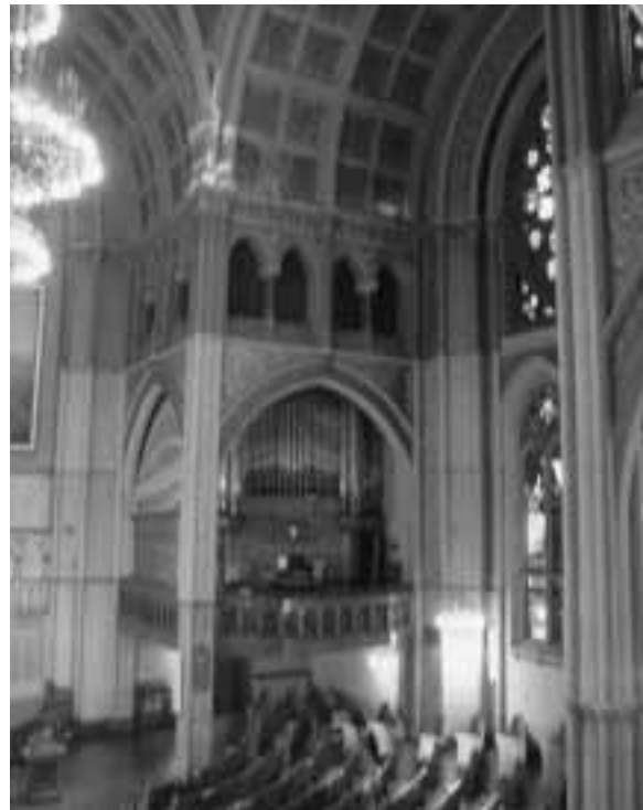
Old First Reformed Church, Park Slope, Brooklyn (1891) features scagliola colonnettes in the clerestory.
