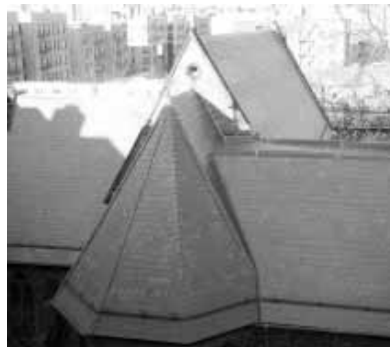
The work in progress and the final result.
