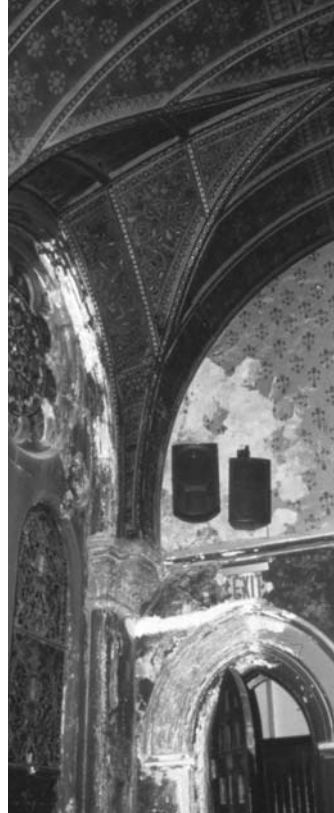
Clockwise: 1. Water-damaged plaster moldings, walls, and arches amidst original decorative painting at Emmanuel Baptist Church. (Trix Rosen) 2. Unstable plaster over a doorway was removed down to brick. 3. Replication of moldings by EverGreene plasterers. (John Favazzo, Li/Saltzman Architects)
