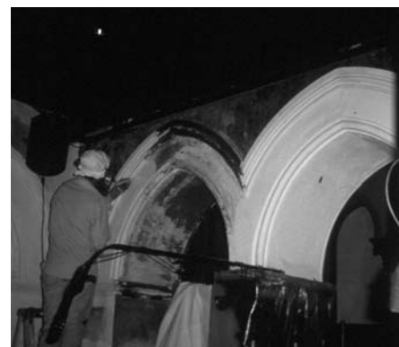
Clockwise: 1. Water-damaged plaster moldings, walls, and arches amidst original decorative painting at Emmanuel Baptist Church. (Trix Rosen) 2. Unstable plaster over a doorway was removed down to brick. 3. Replication of moldings by EverGreene plasterers. (John Favazzo, Li/Saltzman Architects)
