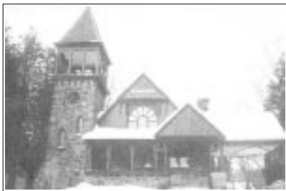
Grace Memorial Chapel in Silver Bay, NY was awarded $4,000 to fund half of an $8,000 masonry repair project. Courtesy of Grace Memorial Chapel
