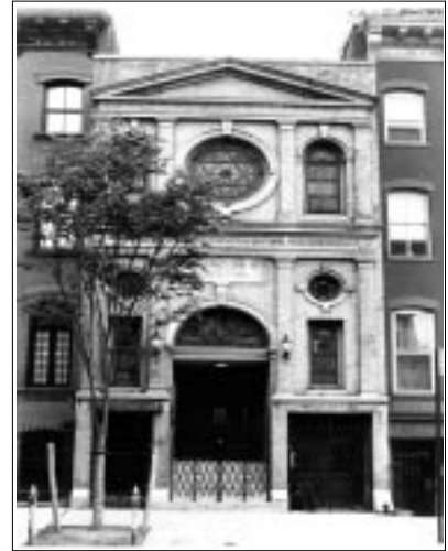
Congregation Darech Amuno, on Charles Street in Manhattan's Greenwich Village Historic District (Architect unknown), was originally a rowhouse dating from 1868; between 1912 and 1917, the building was gutted and renovated as a two story synagogue.
