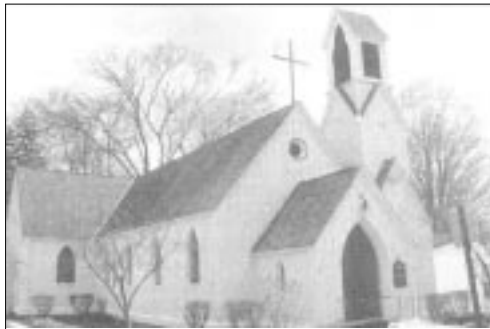
The congregation of St. Thomas's Church in Hamilton, NY was awarded $25,000 to help replace its cedar shingle roof and repaint the building according to the architect's original design. Courtesy of St. Thomas's Church
