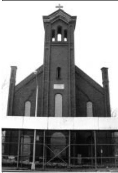
A sidewalk bridge was erected before St. Monica’s Roman Catholic Church in Jamaica, NY. A bridge both provides a workers’ platform and protects passersby from falling debris.
